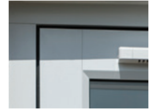
Timberweld jointed sash and outer frame
