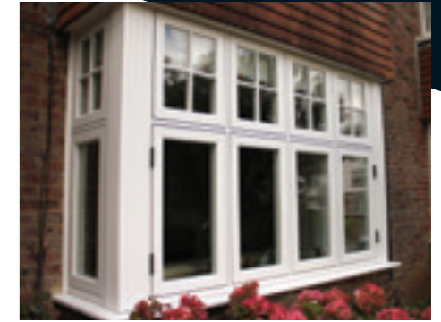
Flush external finishes with equal sightline
