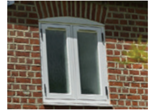
Dummy butt hinge upgrade (Functional butt hinges not available)
